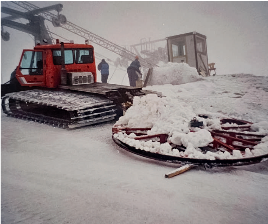
Replacing the rope sheave bearings on the Saxnerjoch
